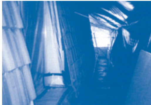
Commercial asbestos removal
